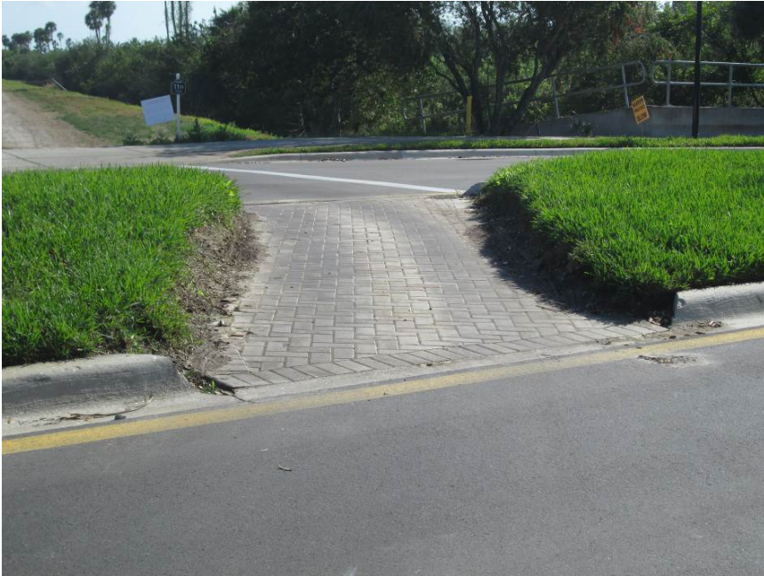
Cart Crossing Stone Harbour Loop viewing south – curb deficiencies.
